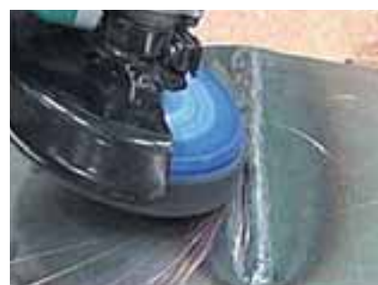
*Removing blue weld discoloration
