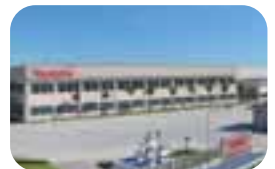
THAILAND Makita Manufacturing (Thailand) Co., Ltd.
